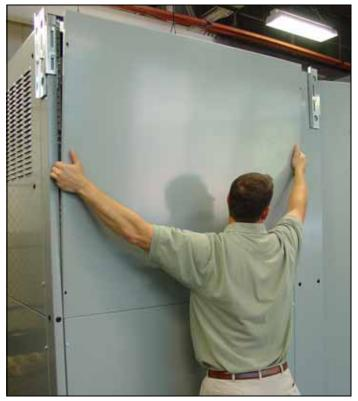
Figure 41. Lifting the Cover Free.
